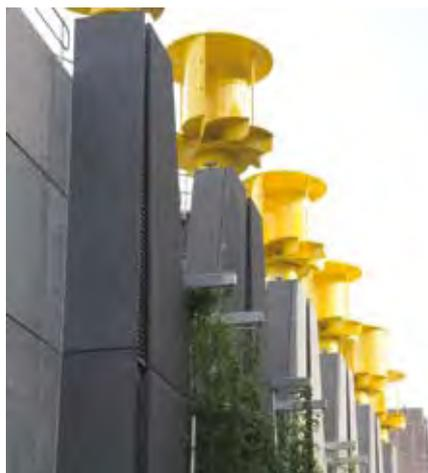
*CH<sub>2</sub> wind turbines for drawing air out of the building*
